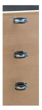
The insert provides perfect protection against scratches from the metal parts, but turned out to be too soft for effective clamping. That actually is no surprise as it has been designed for sound insulation purpose, not to prevent rotation (not a reasonable use case for pipe installation anyhow).
